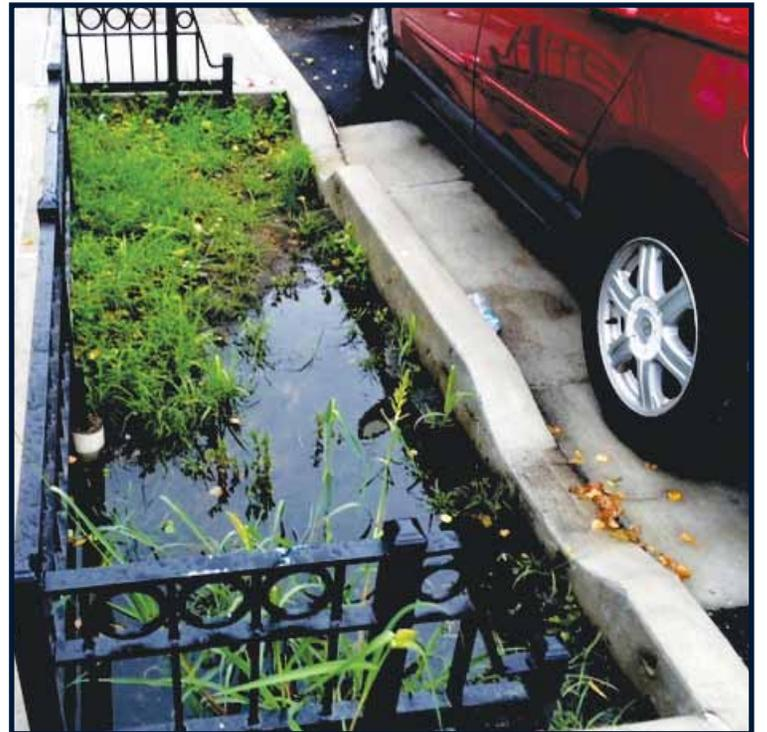
Pictured above is what happens to a bioswale in an area with a high water table the water remains in pit.
